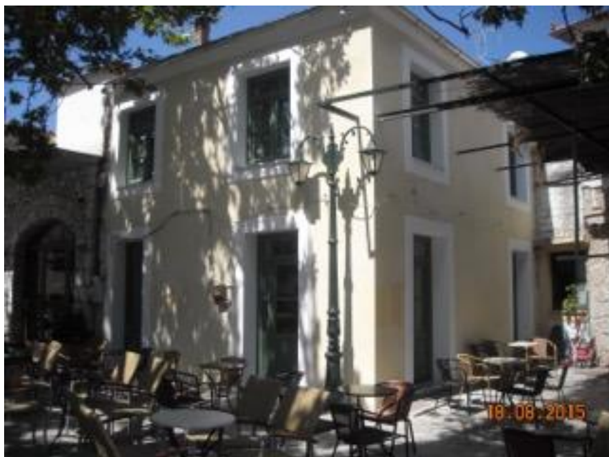
The building after its restoration
